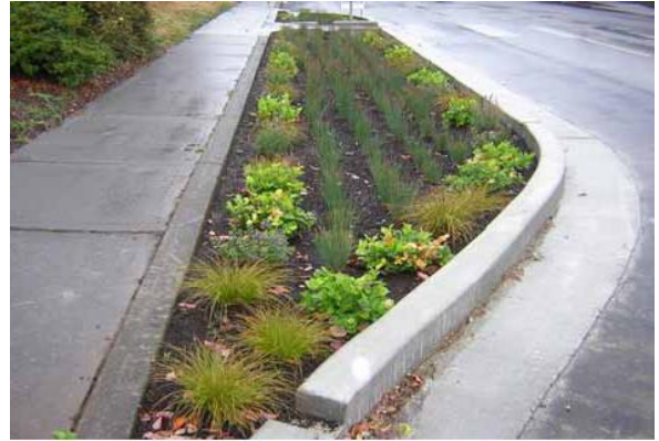
Some cities use storm water planters to manage street runoff and improve water quality.
