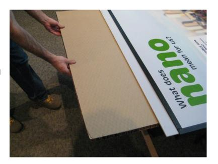
Once the graphic is upright make sure that the top edges of the graphics are being overlapped by the metal frame: there is a certain amount of flex to the frame and occasionally the top edge of the graphic will pop free during installation. Pressing the top edge of the graphic in place and pulling down firmly of the top crosspiece of the frame will remedy this problem.
